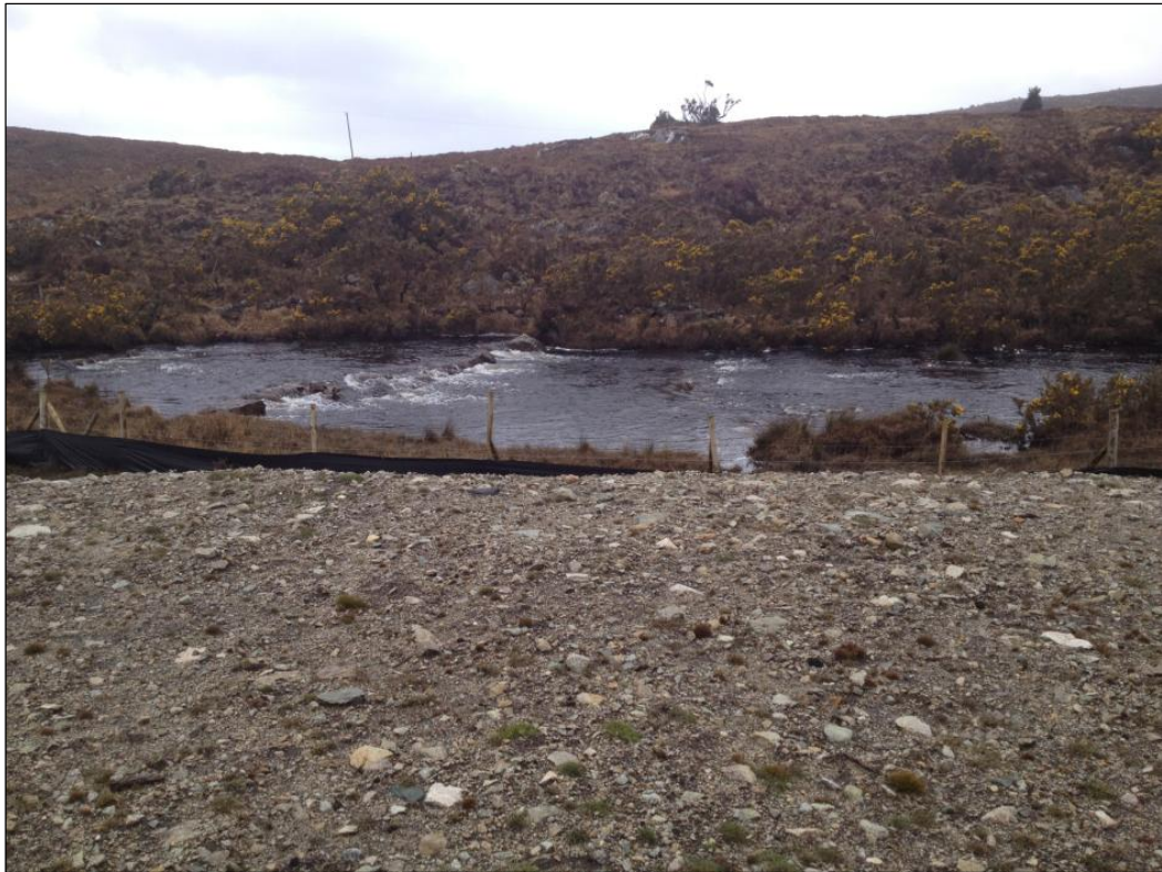
Plate 7.3-A Existing Silt Fence between Shannapheasteen Stream and the quarry haul roads
