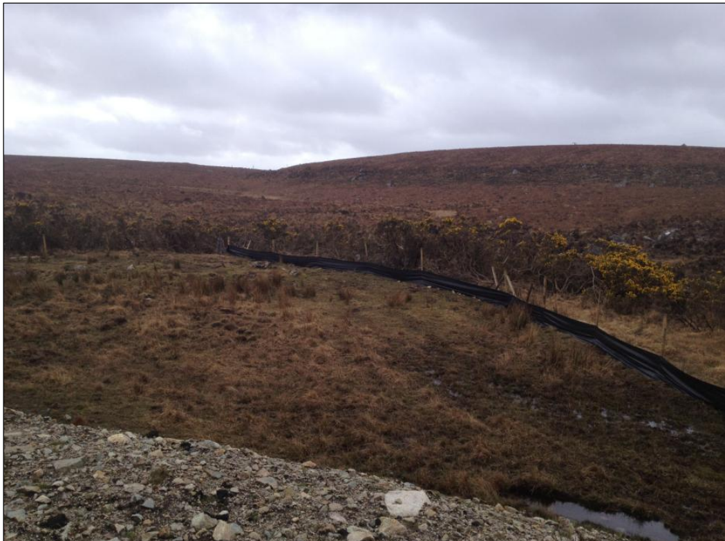
Plate 7.3-B Existing Silt Fence between Shannapheasteen Stream and the quarry haul roads
