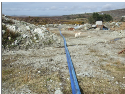
Plate 3.7 Hose running from extraction area to vegetation polishing filter
