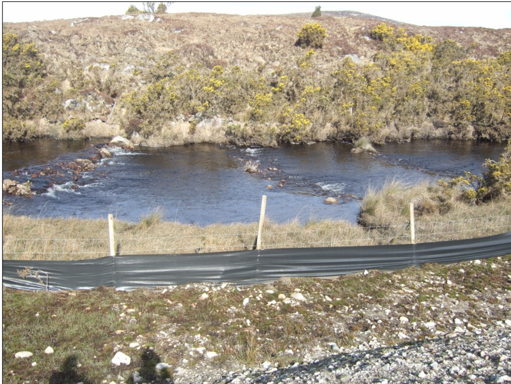
Plate 3.8 Silt fence embedded in ground and attached to wooden stakes to protect river
